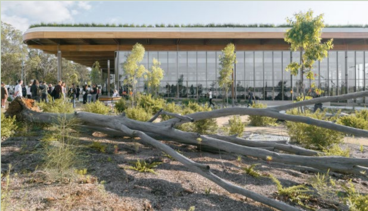
AMRF First Building - Image: Hassell / Vinchy Wu
